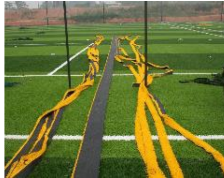
Figure 18: Installation of in-laid lines
