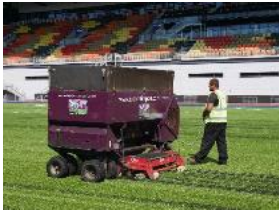
Figure 19: Installation of performance infill
