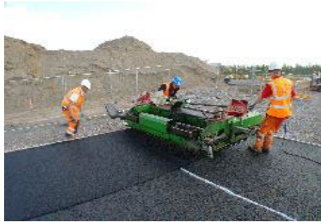
Figure 14: Installation of shockpad
