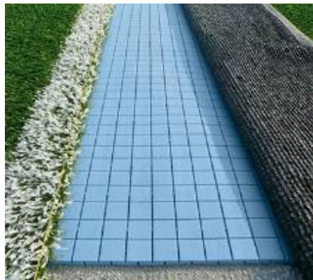
Figure 9: Image of shockpad installed in a synthetic turf system
