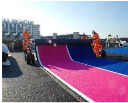
Figure 16: Installation of carpet
